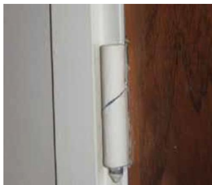
Figure 5 Rising Butt Hinge
